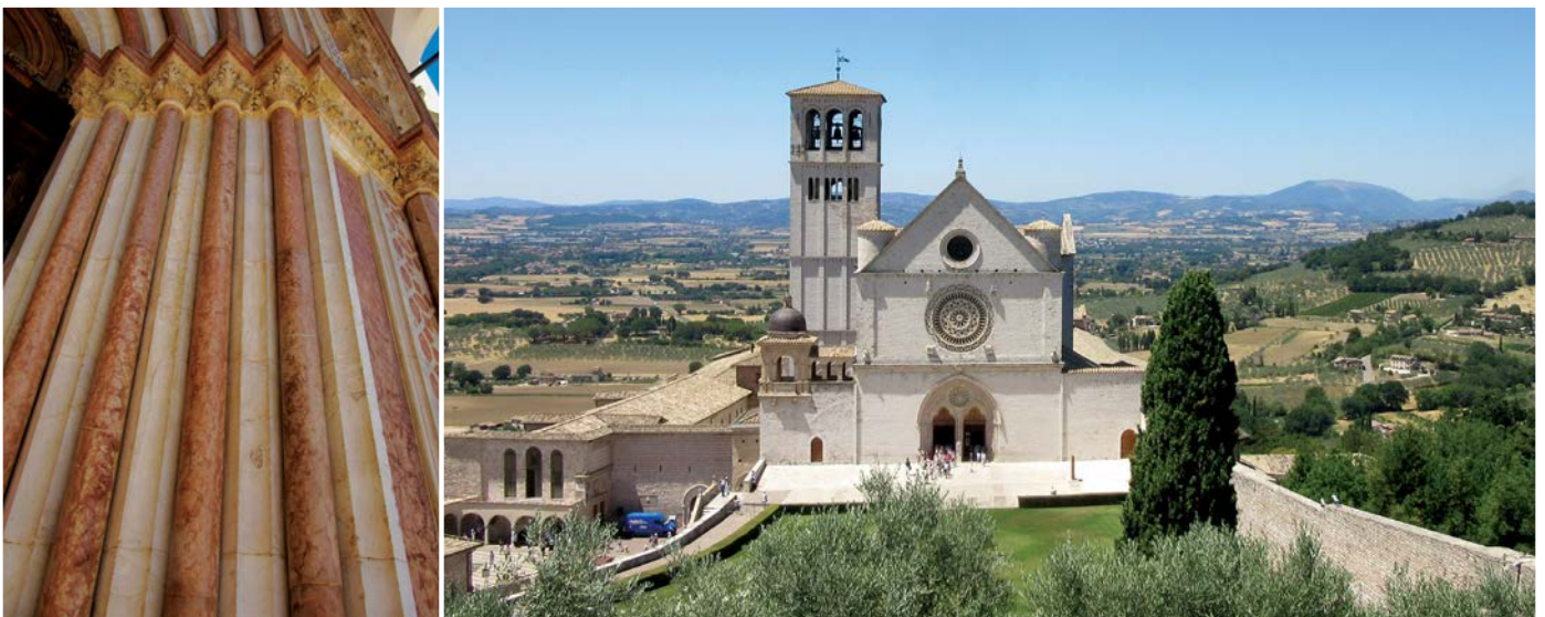
The Basilica of St. Francis in Assisi, about 40 kilometers west of Monti Sibillini National Park, has a distinctive pink color because it was built from the Scaglia Rossa limestone.
