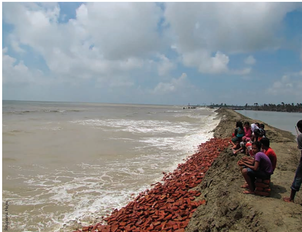
Coastal embankments in the Indian part of the Ganges-Brahmaputra Delta region protect low lying land and vulnerable households.
